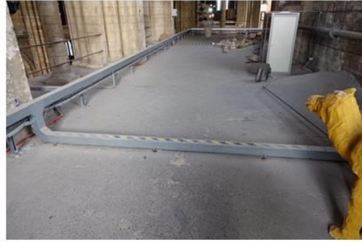
Example of trip hazards on the Triforium level
