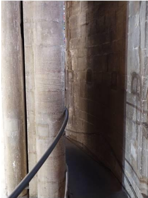
Narrow, curved passage way around the Apse Chapel
